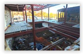
The new water supply for the sprinkler system was tied into the water main in 90th street last week and steel will be nearly completed. This week, they plan to pour the 2nd floor deck and begin the masonry work for the elevator shaft.
