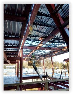
Decking on the roof and second floor is being installed.
